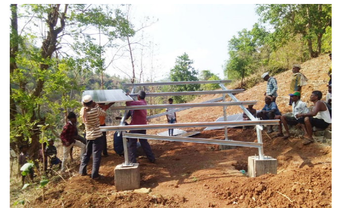
Solar panel installation for water lifting
